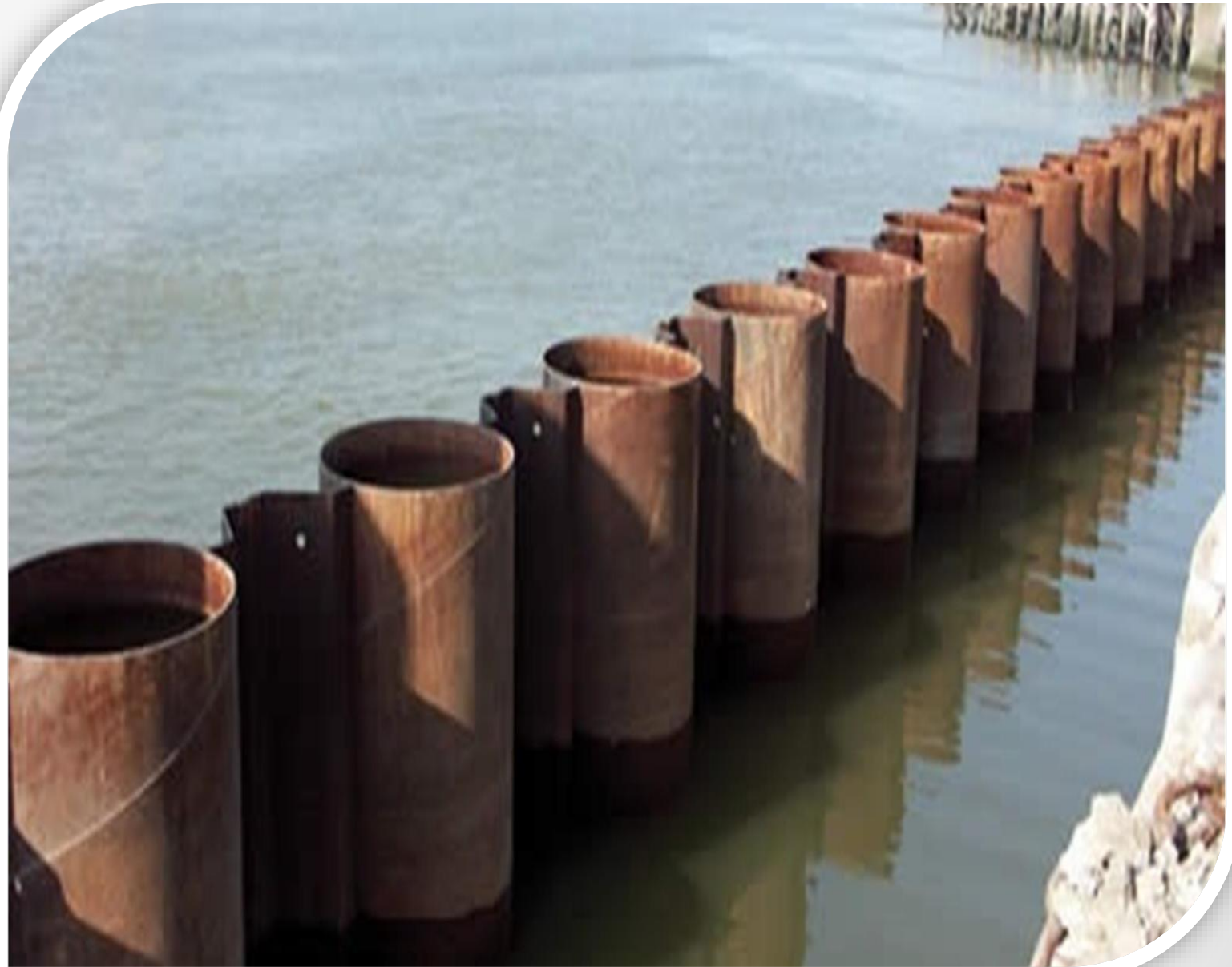
Representation Image of Combi wall ( Tubular & AZ)
