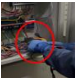
① Connect low-voltage clamp
