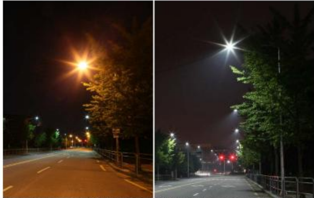
Comparison between HPSV (left) and LED (right): While conventional technologies can meet the key lighting factors (luminance, uniformity, glare, surround ratio, color rendering index), LEDs meet these at more desirable levels, making it more pleasing to the eye, as evident in the pictures above.
