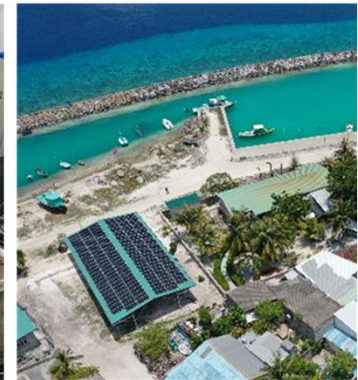
Solar PV at the project site
