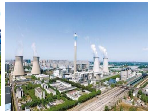
The first coal-fired power plant meeting ultra-low emission standards
