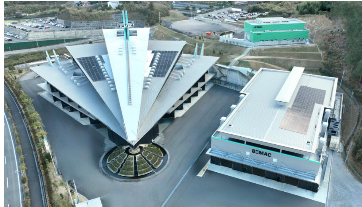
Imabari Head Office / Mirai Factory
