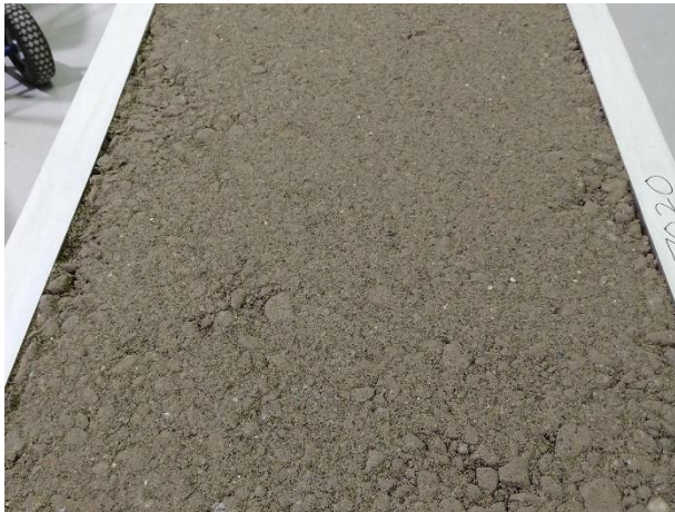
Surface after compaction
