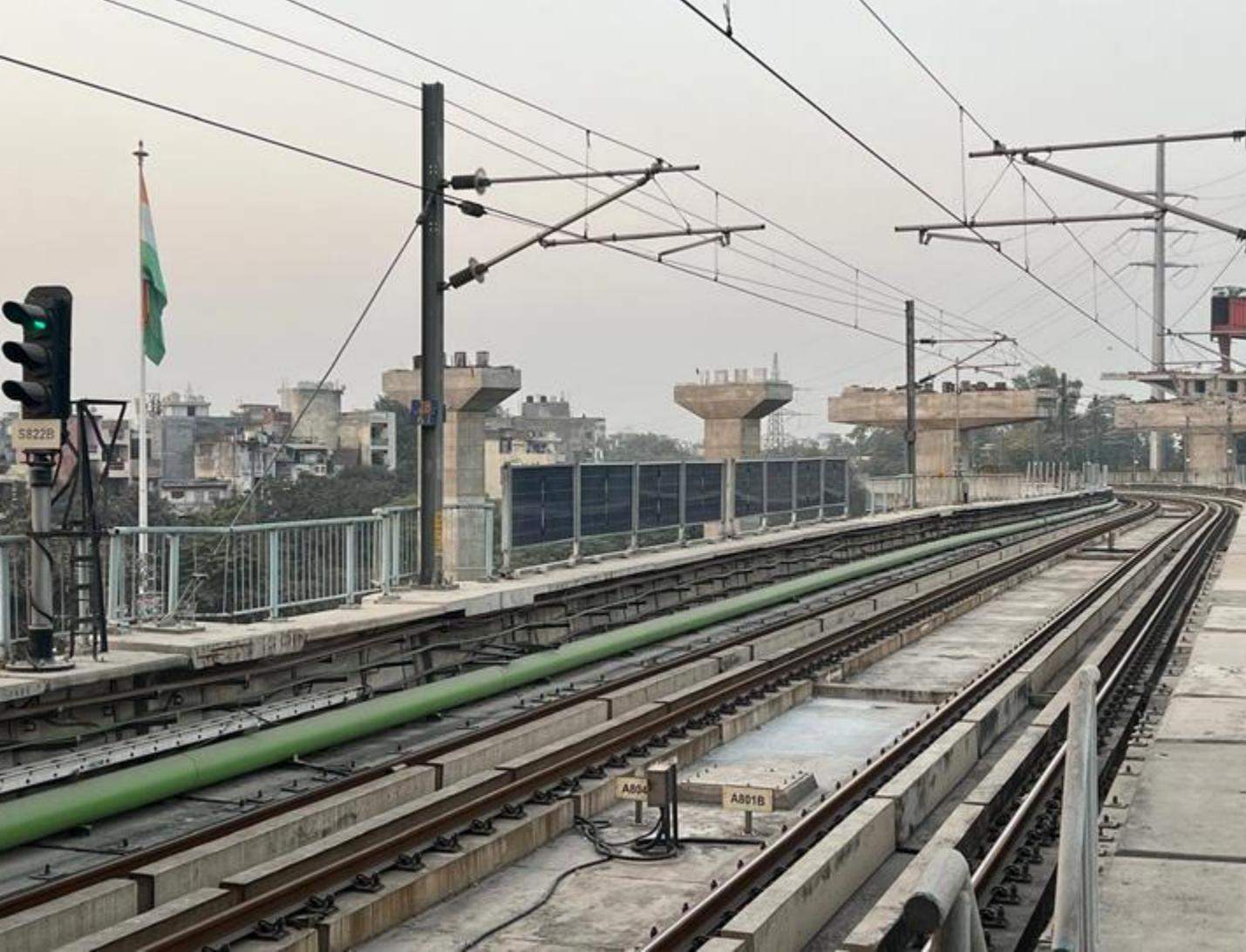
Delhi Metro is currently installing a first-of-a-kind vertical PV array using bifacial modules on an elevated viaduct at Okhla Vihar station in New Delhi.
