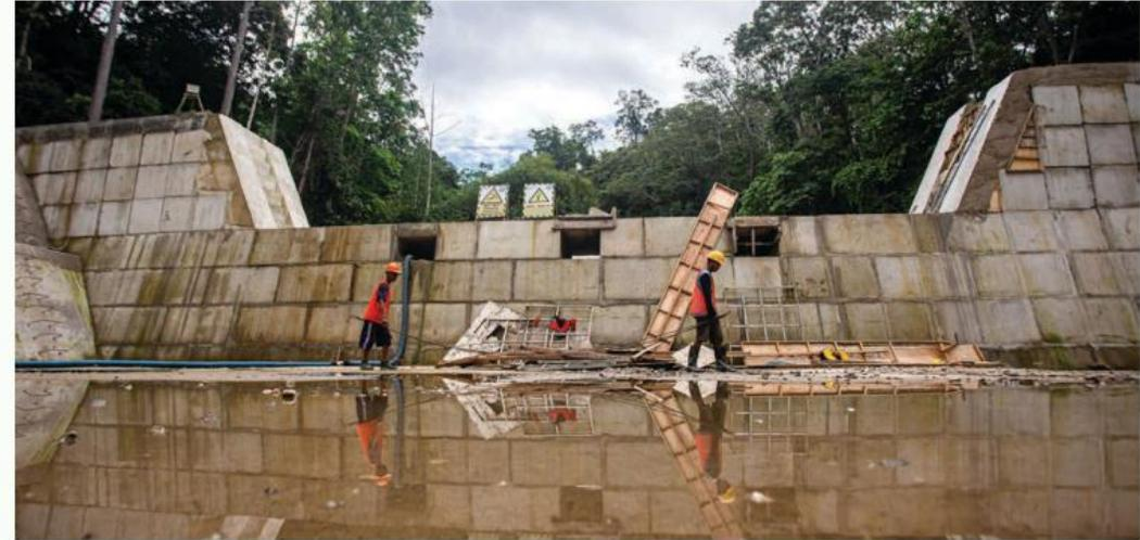
ADB Indonesia: Emergency Assistance for Rehabilitation and Reconstruction Project (52316-001). The project supported the resilient reconstruction of the Gumbasa irrigation system in Central Sulawesi following the 2018 earthquake and tsunami.
