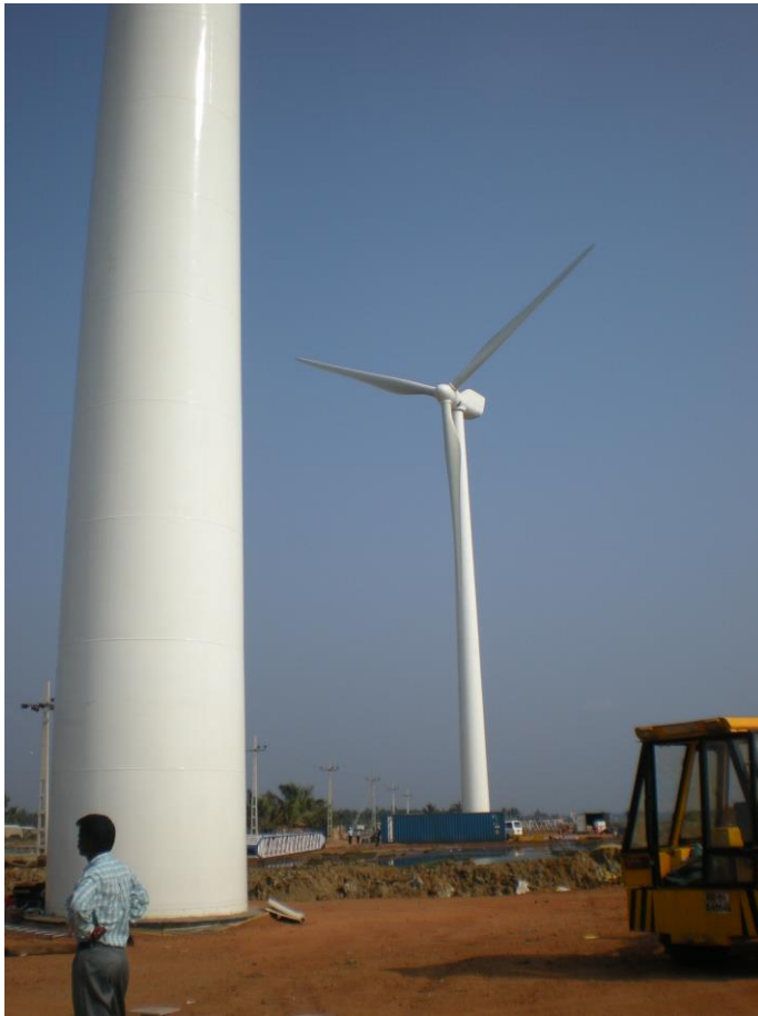
Puttalam 2010: Completed 1.25 MW wind turbine
