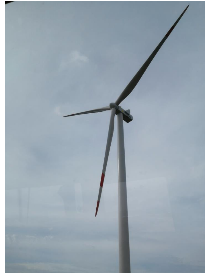
Mannar 2020: Completed 3.4 MW wind turbine
