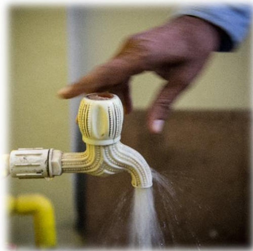
Water Supply, Sanitation, Sewerage
