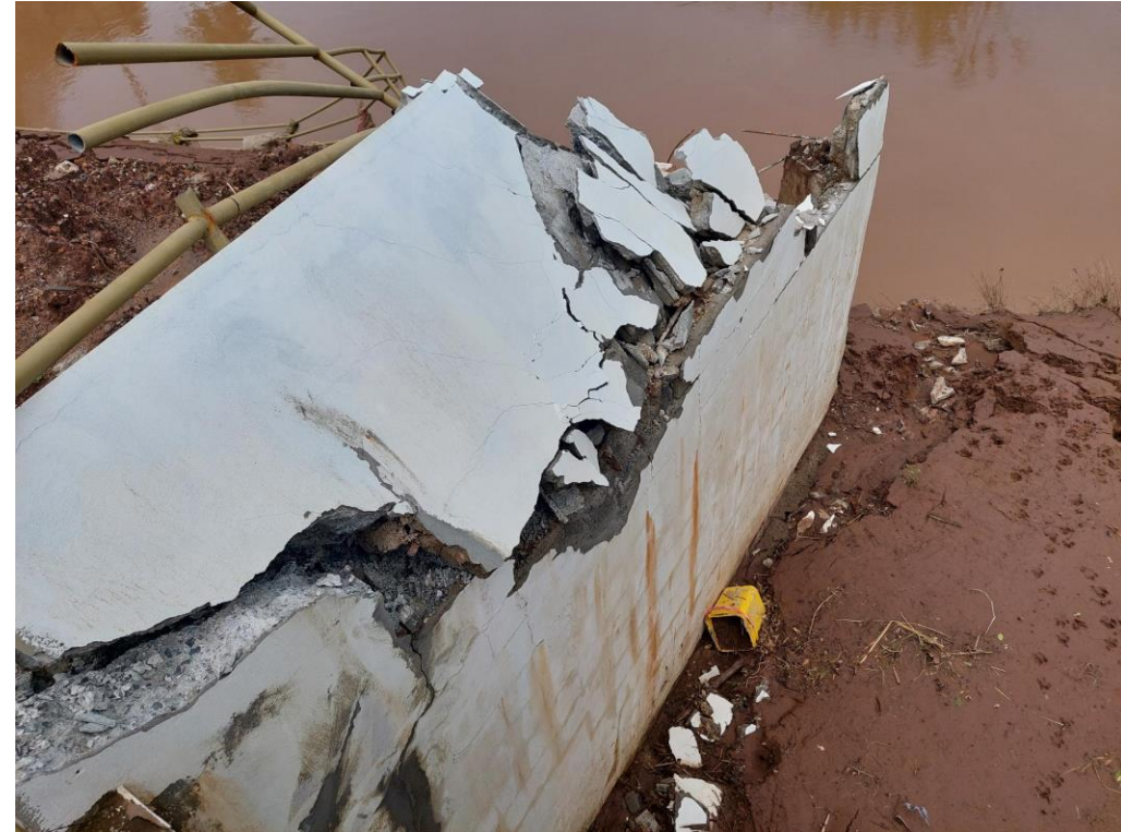
Damage to the earthworks due to the retaining wall collapsing into the river
