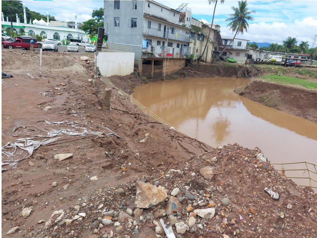
Damage to the earthworks due to the retaining wall collapsing into the river
