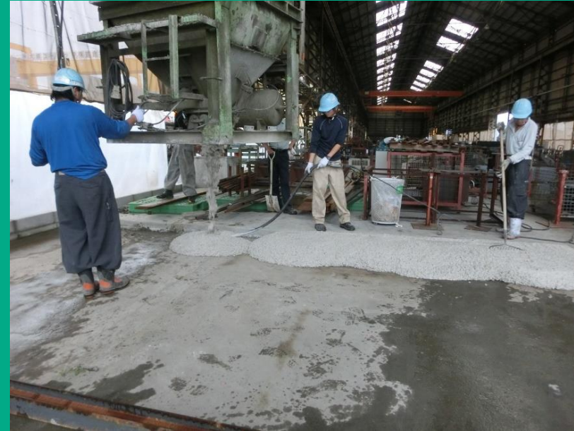
Bucket Placing
