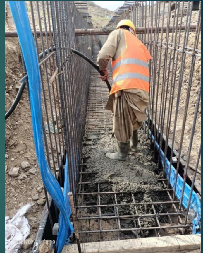
Worker wearing PPE's
