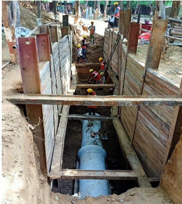
Sewer Line shifting
