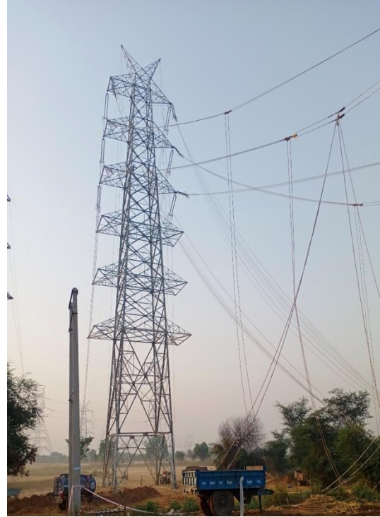
Shifting of EHT Transmission Electrical Lines 400 kv at Panchgaon
