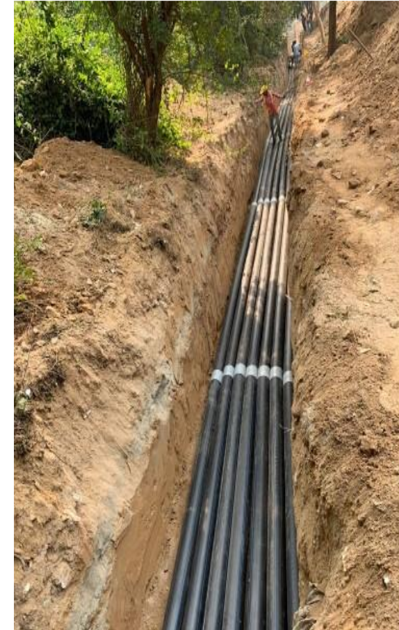
Laying of 11 kv U/G Cable at Manesar
