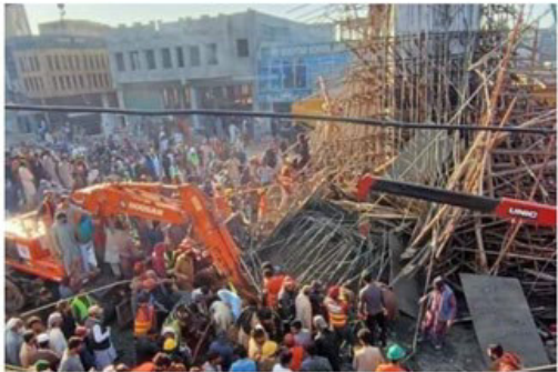
Above: Heavy vehicles were reportedly allowed through the site while work was underway
