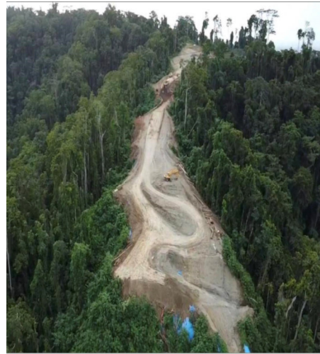
LOT 2-2 Earth works
