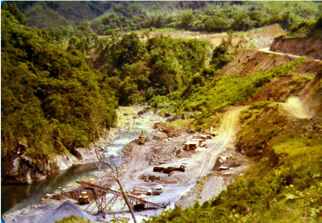
Power station site – 1979
