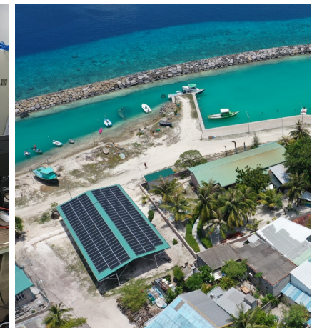
Solar PV at the project site
