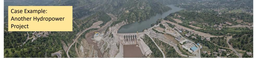
**The Project:** A run-of-river scheme HPP which generates power by diverting flow short-cutting a bend in the river.
