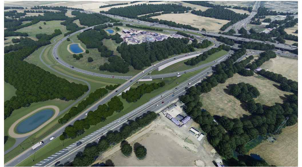
Atkins M25 A12 interchange J 28 – improved the water environment
