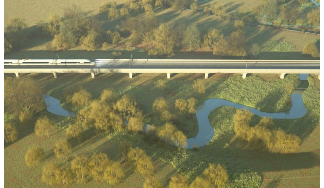
HS2 Cherwell Valley Viaduct – allowing free flow of flood water
