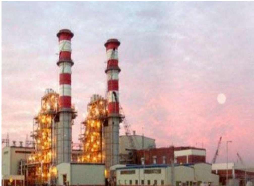
Picture: Meghnaghat Power Project
