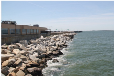
Sea Wall and Riprap
