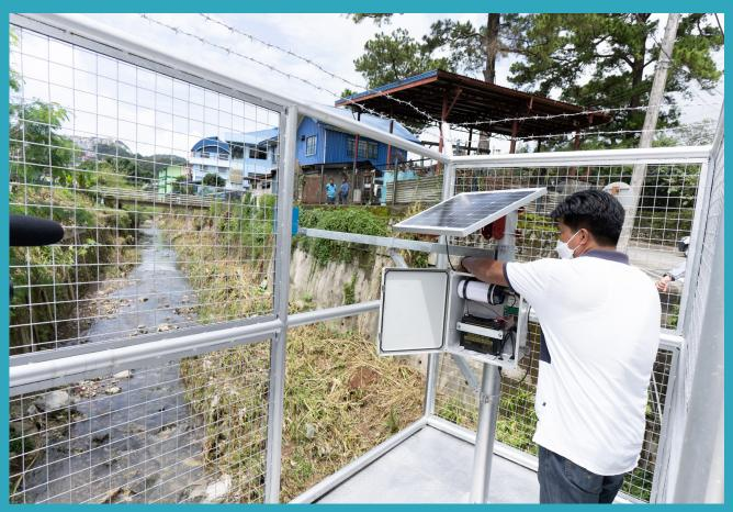
**Figure 40: Monitoring station at Fergusson Bridge. The station was constructed as part of the project in 2022.** Source: Ramboll
