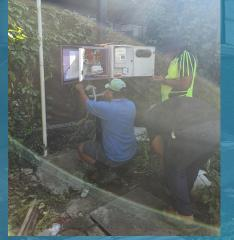
SWA team installing smart control panel for better flow controls and data logging
