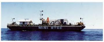
The first closed cycle Mini-OTEC plant to produce net power (15 kilowatts) at Keahole Point, Hawaii, in 1979
