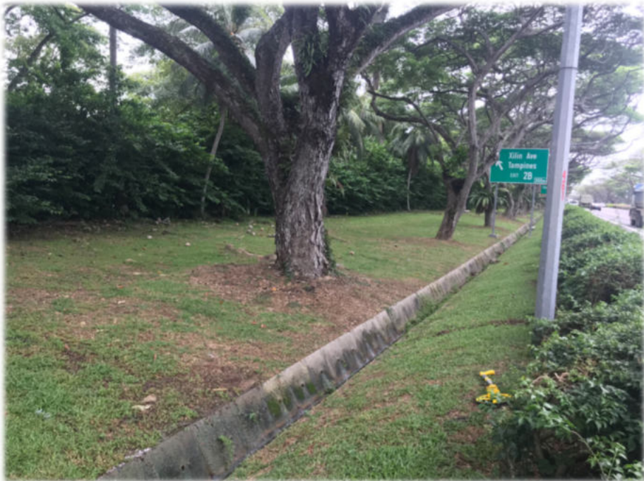
No visible signs of leakage
