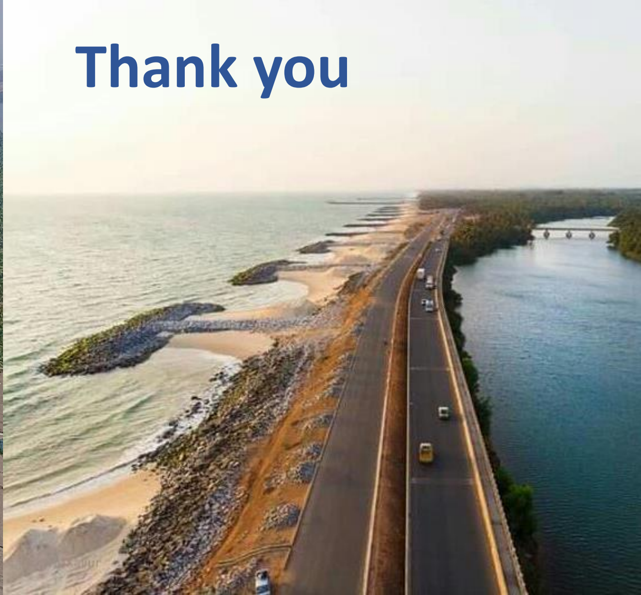
Maravanthe sub-project, Groynes and sand re-distribution
