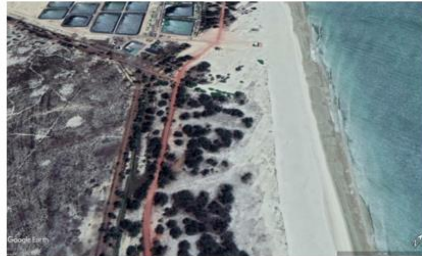
A low-lying section of the Bao Ninh to Hai Ninh coastal road. Source: Google Earth
