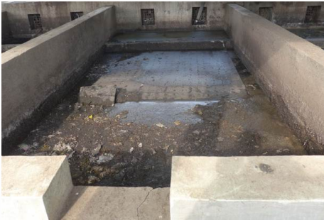
Solids Separation Chamber
