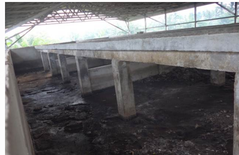
Sludge Drying Bed
