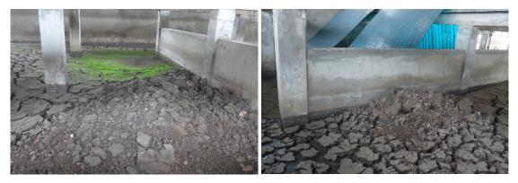
Figure 52: Dry Sludge Accumulated in the Sludge Dying Beds at the Talang Bakung IPLT
