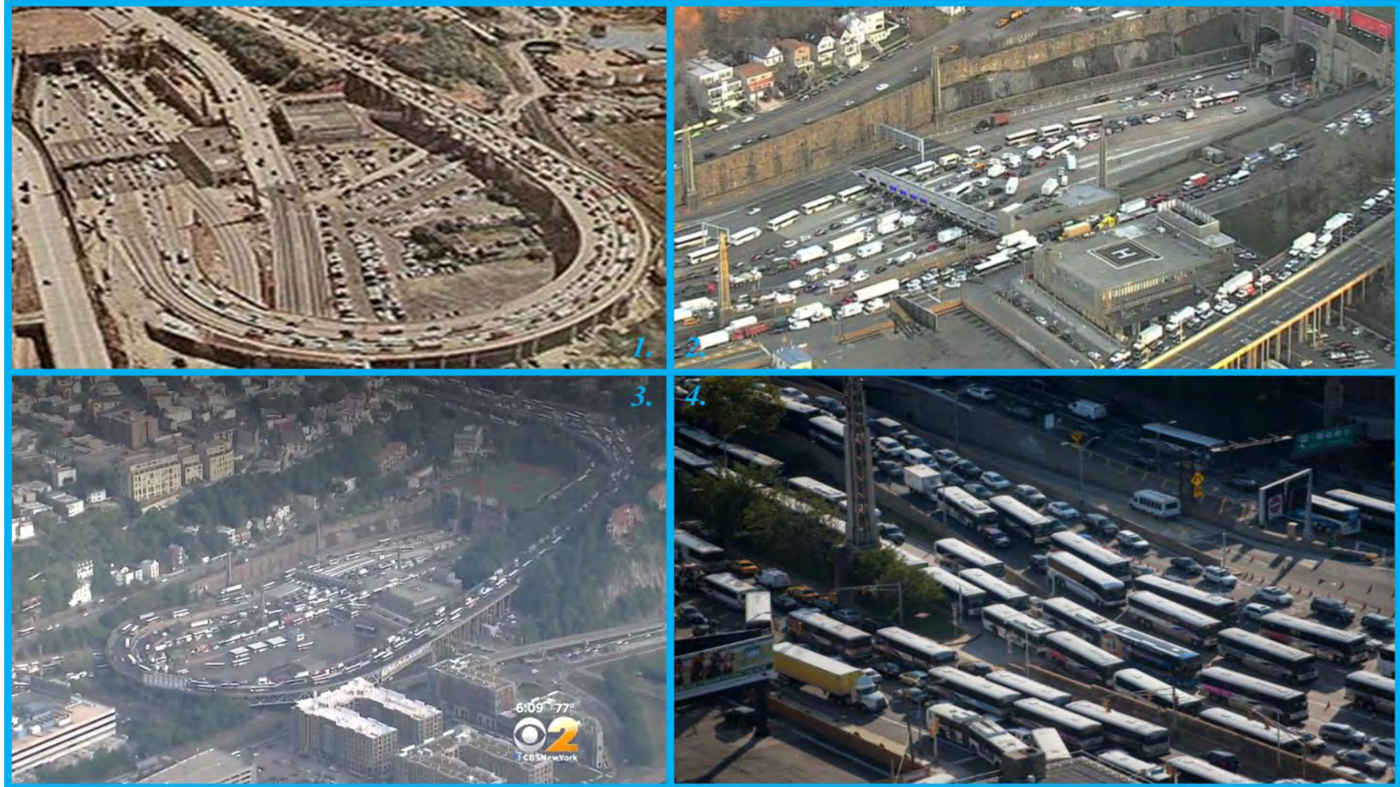
Aerial footage on Lincoln tunnel (NY-NJ bidirectional)
