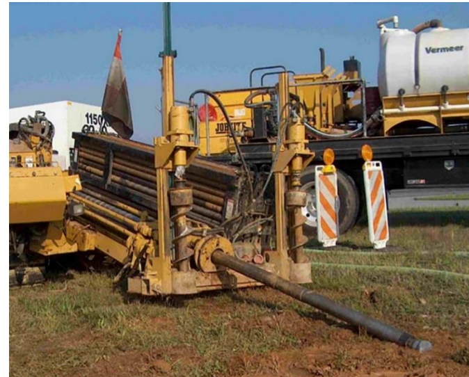
Horizontal Directional Drilling: \Phi from 40 to 1200mm
