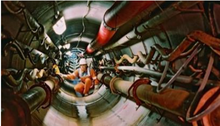
Microtunneling: \Phi from 500 to 3500mm
