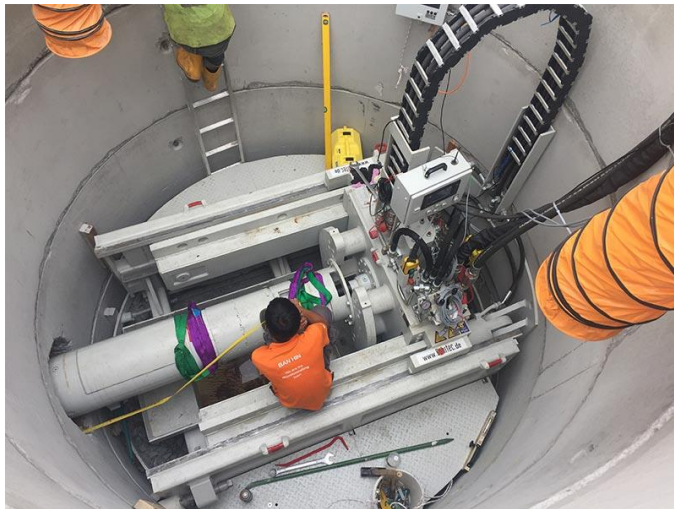
Auger drilling: \Phi from 250 to 1500 mm
