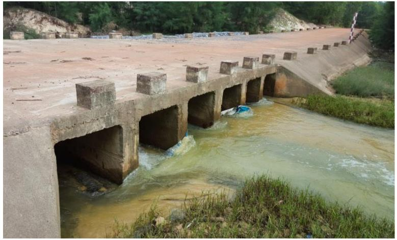
Bao Ninh to Hai Ninh coastal road, Quang Bing Province. The proposed structures are at risk from (1) high-intensity rainfall and insufficient flood conveyance through culverted sections; as well as (2) flooding and/or damage by storm surge-tide-wave interactions with sea level rise.
