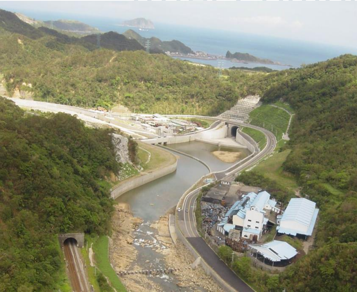
Bird View of Entrance
