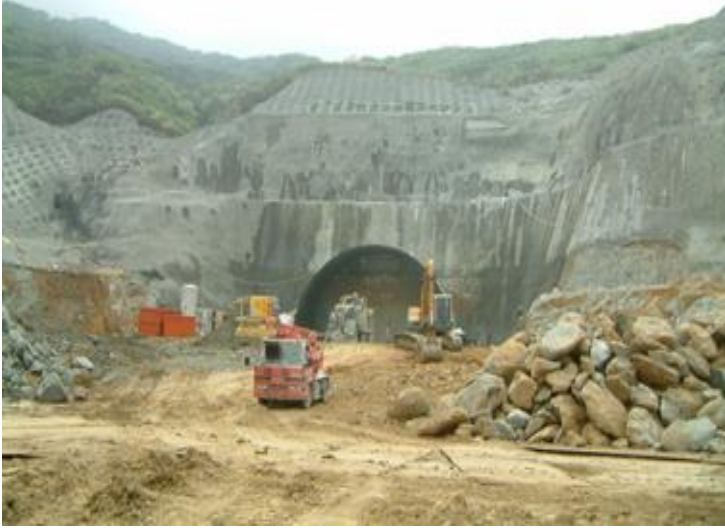
Mar,2003-Before the tunnel excavation
