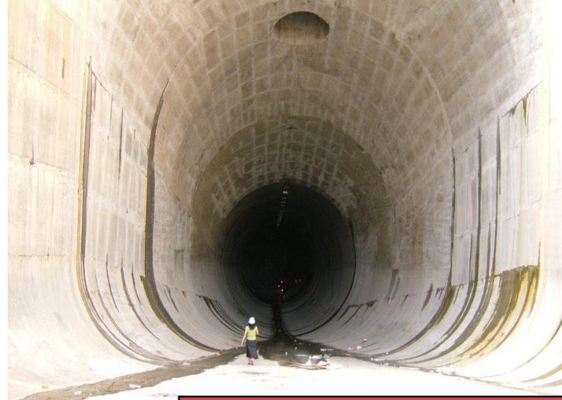
May,2003-Completion of tunnel
