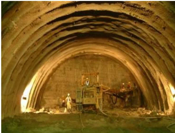
May,2003-The tunnel excavation
