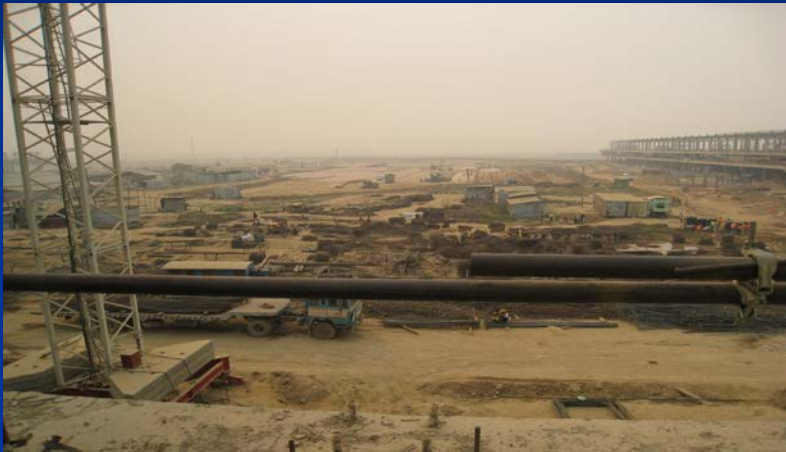
Delhi International Airport Construction Site
