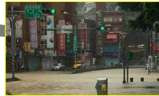
Urban storm sewer
