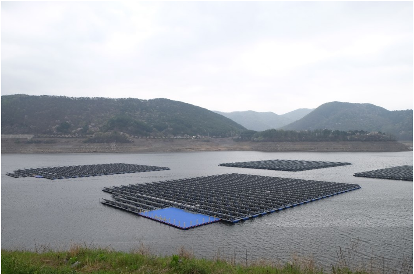
Image: Distributed renewable sources come in all forms including floating solar panels for applications in land constrained regions. Program Participants viewed the floating solar panels on Day 2.
