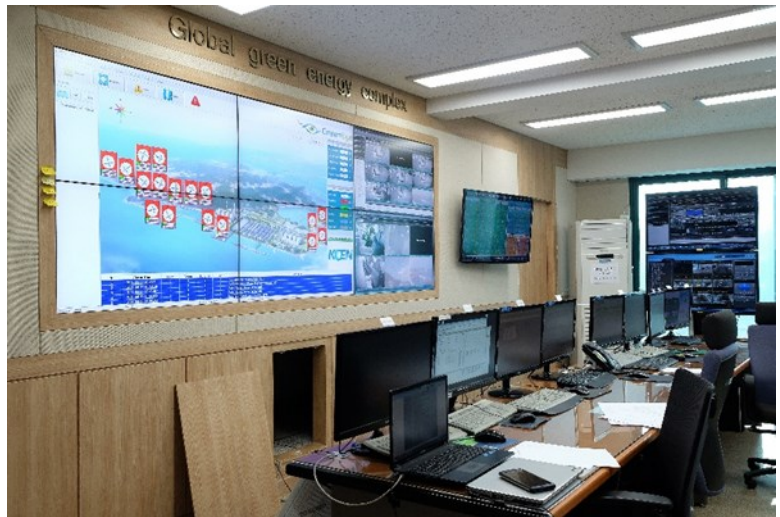
Image: Situation room for KOEN's 4MW wind power ESS commercial project with dashboard monitoring of individual wind turbine health and status.
