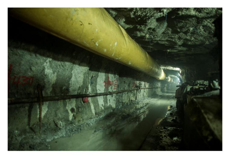
Water tunnel – 25.9 km, 12.9 m2, Design Discharge – 6 m3/s, overburden max – 1,181.7 m
