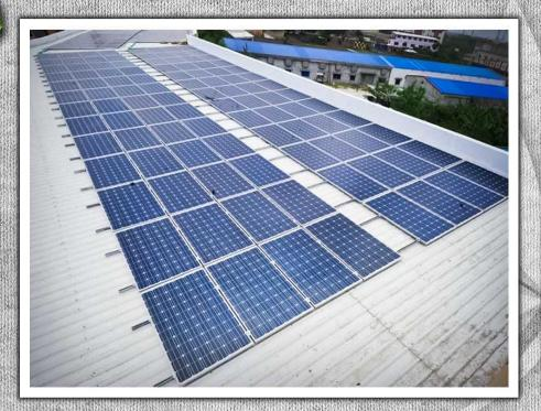
A 65 KW capacity solar power plant with highly efficient mono crystalline panels has been installed in this factory. It will produce at least 110 mw/ hour energy every year which will meet at least 13% of total power required.
