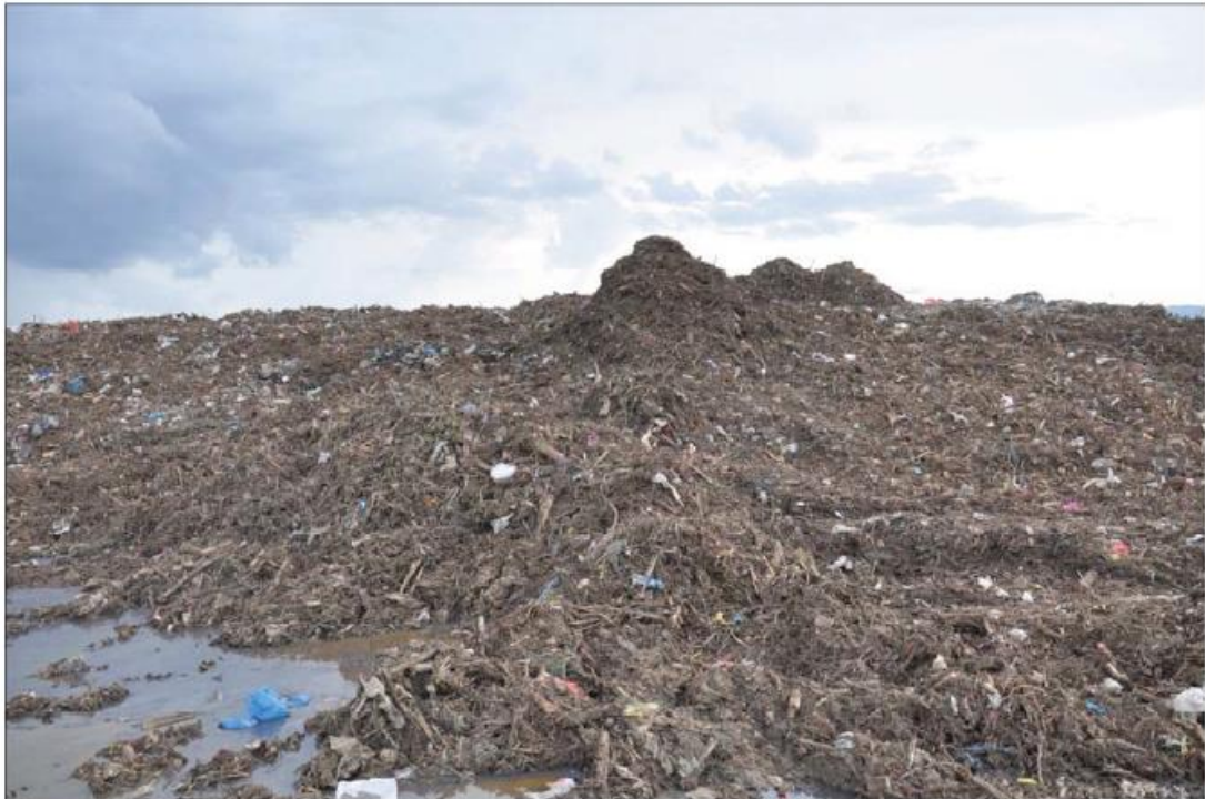
Figure 7 Application of unutilized compost as regular cover in Gampong Jawa Landfill, Banda Aceh, Indonesia.
