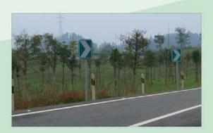
The new design includes updated safety barriers, realignments, paved shoulders, improved delineation and curve markers, enhanced skid resistance and traffic calming
