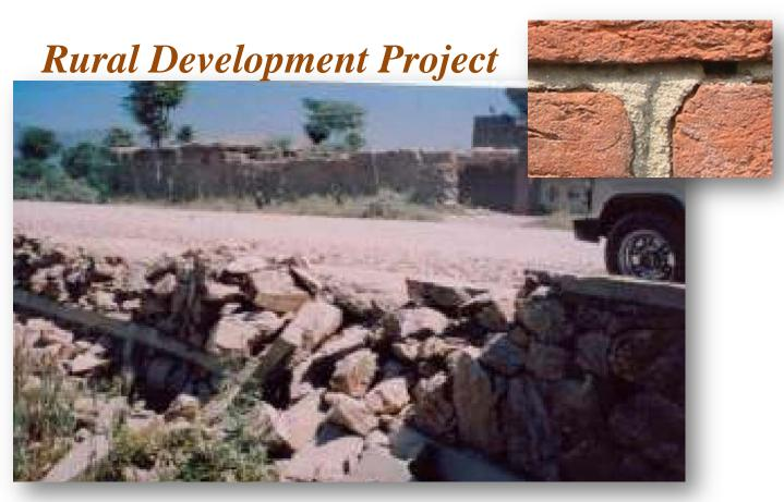
Poor workmanship of a retaining wall, causing collapse – lack of mortar
