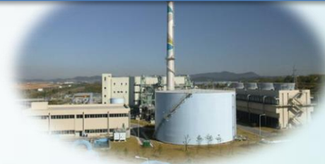
50MW Landfill Gas Power Generation
