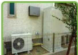
Eco Cute (370L) CO2 Air to Water Heat Pump
