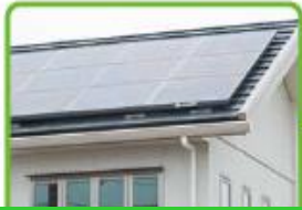
Solar panel (3.2 kW)
