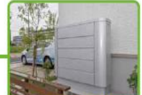
Home battery (5kWh)
