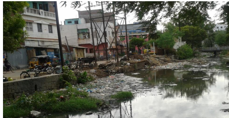
Wastewater flows into tanks from areas with no sewerage infrastructure
