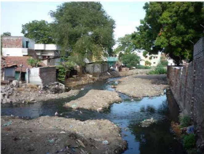
Figure 27 – Many slum areas are built on land along rail and rover corridors and experience multiple vulnerabilities. Water is drawn from channels which are polluted by raw sewage.
