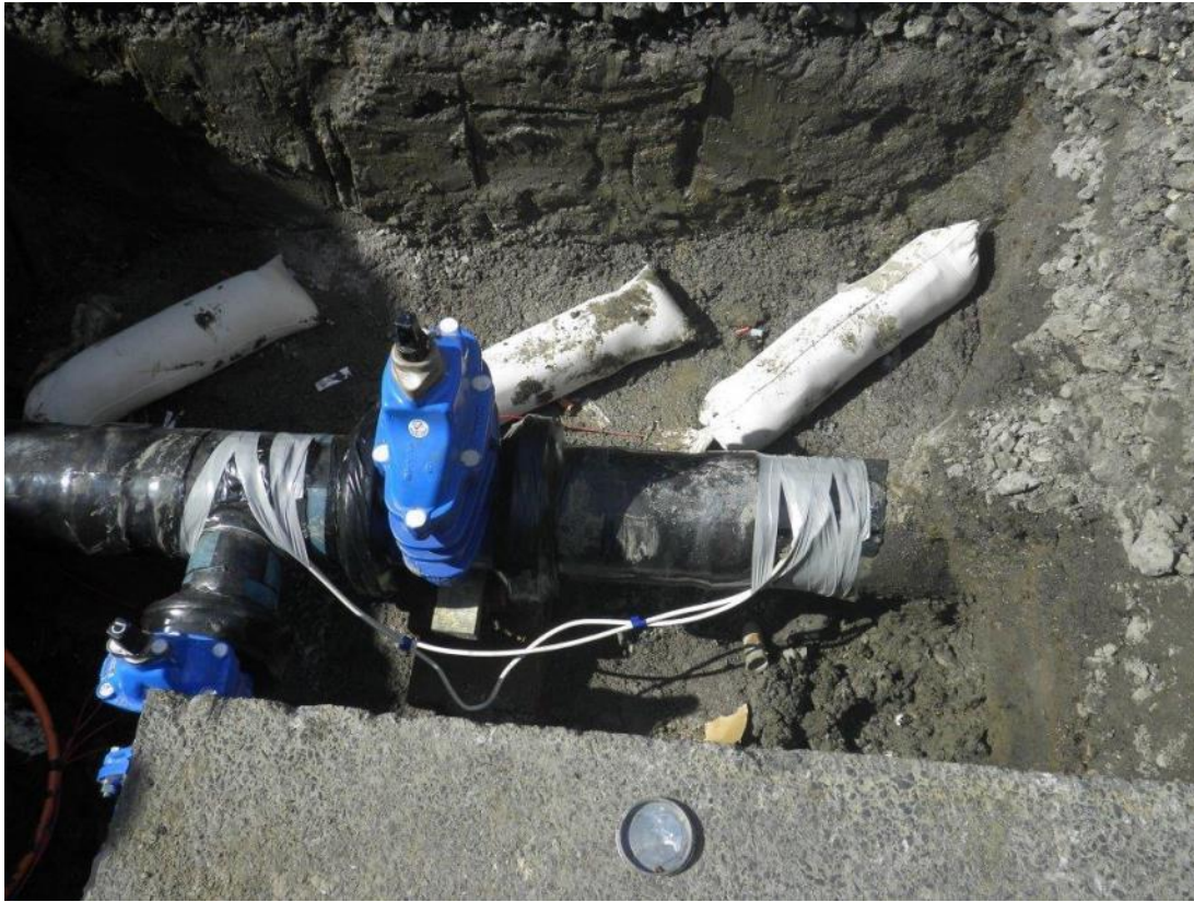
Installation of cathodic protection
