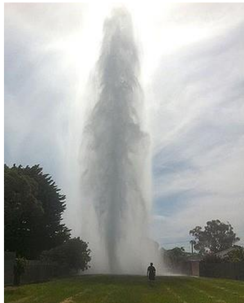
Air valve failure 28/10/2012
