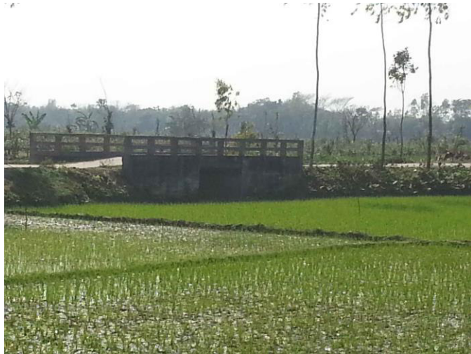
Figure 5: A rural road with a culvert in Narayanpur Union Parishad of Belabo Upazila in Narsigndi constructed under RIIP-2 of LGED. Photo taken during field visit on 20/02/2013.
