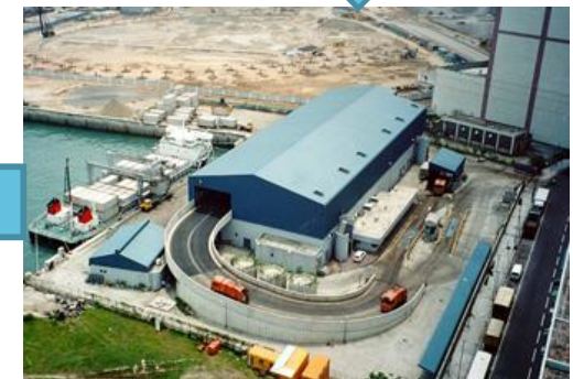
Refuse Transfer Station
