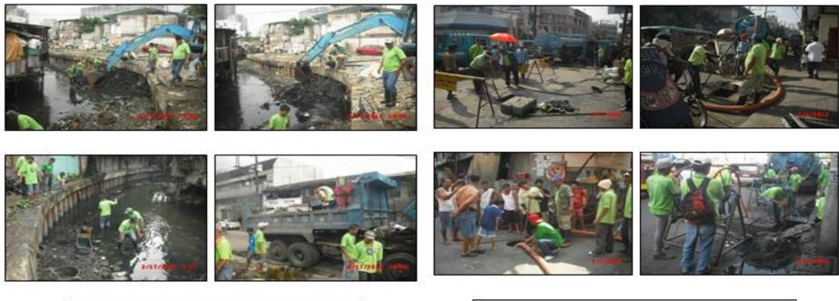
DREDGING/HAULING & DISPOSAL OF SPOILS DECLOOGING OF DRAINAGE SYSTEM USING SRECO, VACUUM TRUCK & SEWER JET
